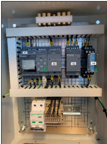
Plugs inside Insulation guard
