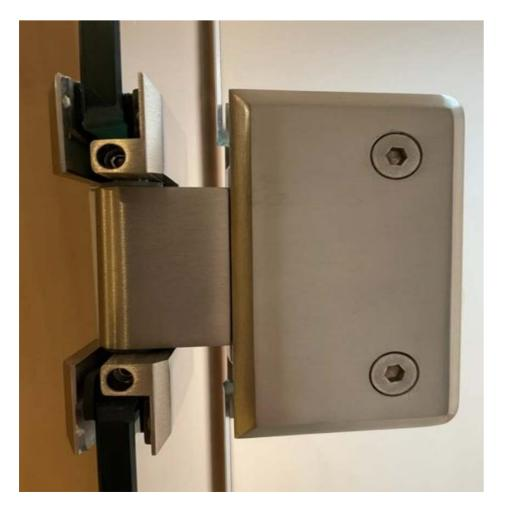
3 The remaining two hex-screws are located on the spine of your hinge - visible only by opening the door. These screws can be tightened by hand using a 2.5mm allen key.
