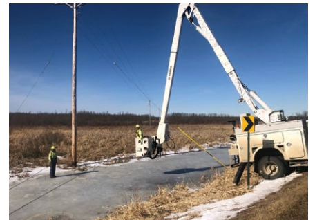
Linemen stringing fiber to Springsteel Island
