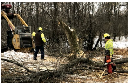
REC crew clearing power line right of way
