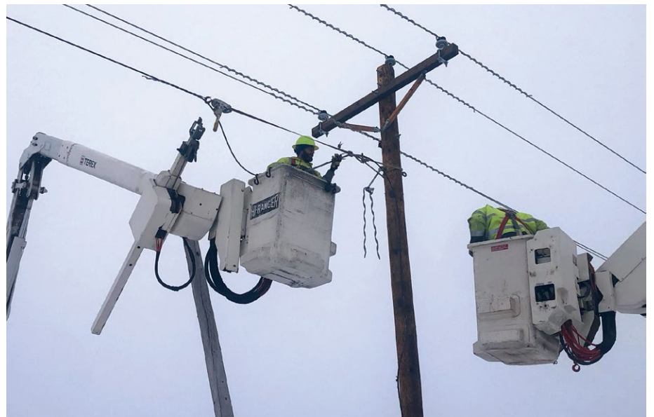
Linemen stringing fiber to Springsteel Island
