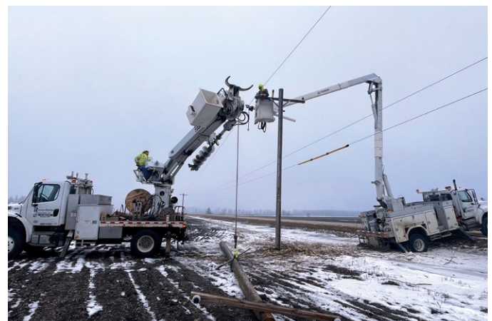
REC line crew rebuilding two-phase power line in Stokes township
