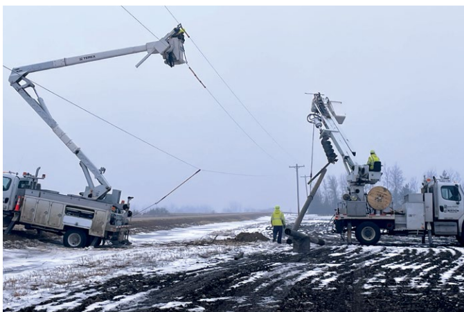
REC line crew rebuilding two-phase power line in Stokes township
