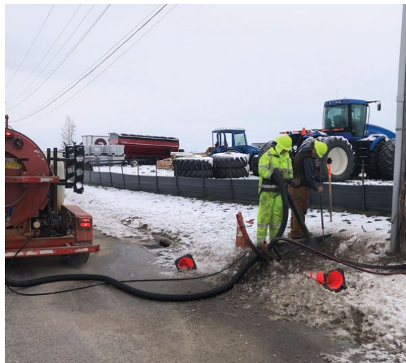
Linemen using the vacuum trailer to locate underground wires
