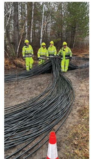
Line crew assisting NorthStream Fiber in installing fiber-optic cable near Warroad
