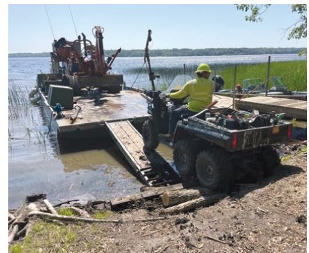
REC linemen loading equipment to be transported onto the islands
