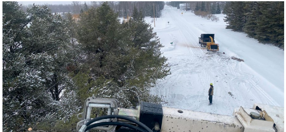
REC crew cutting trees out of power lines
