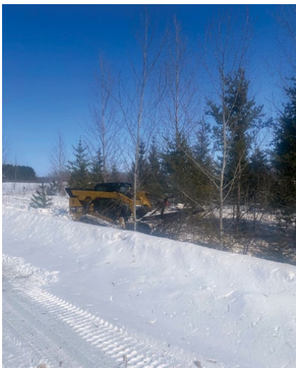
REC crew mowing brush in the power line right of way
