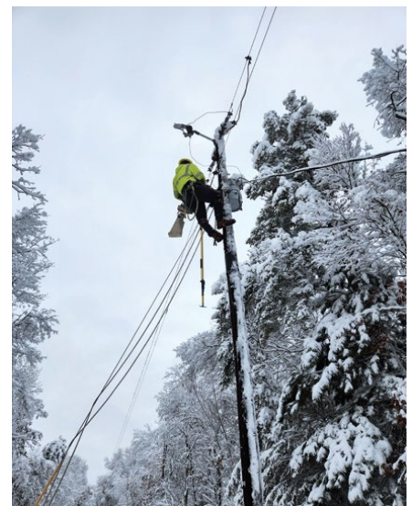
Luke Holland replacing a cutout.
