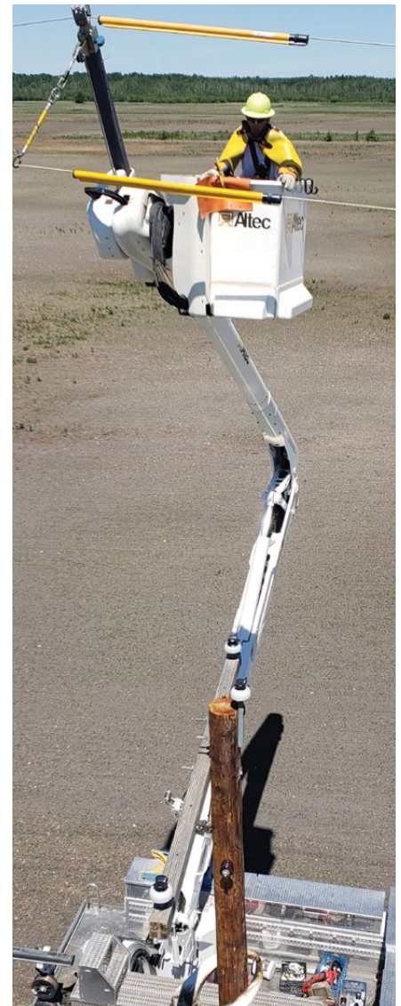
Justin Olson pulls away energized conductors while changing out a pole.
