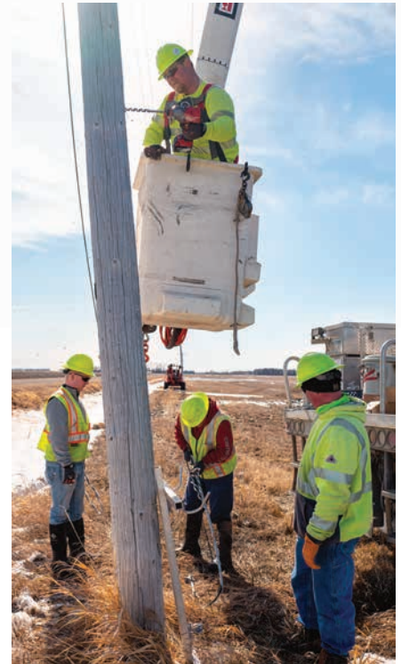
REC’s line crew prepares a stretch of fiber at a future splicing point along the network path northwest of Roseau, Minn.
