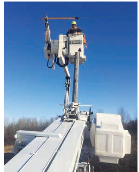
Neal Vatnsdal tying in a new single-phase power pole.
