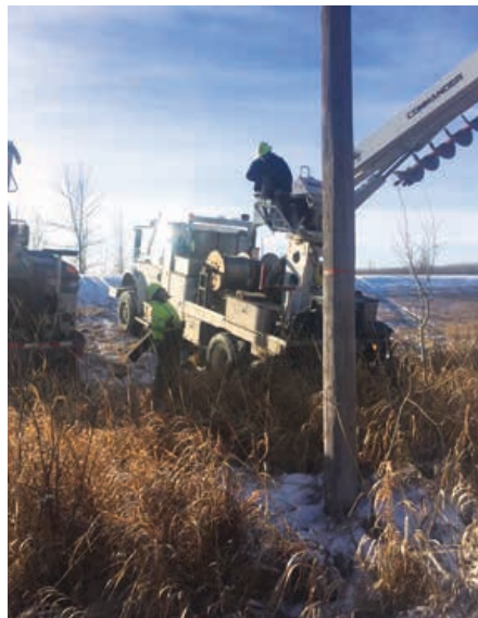
Jedd VonEnde on the digger derrick and Ross Nelson on the ground change out reject single-phase poles.
