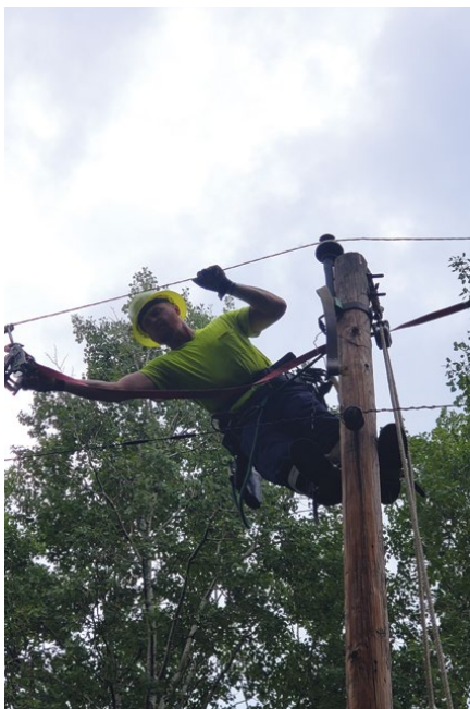
Dillion Thompson repairing a power line south of Four Town.
