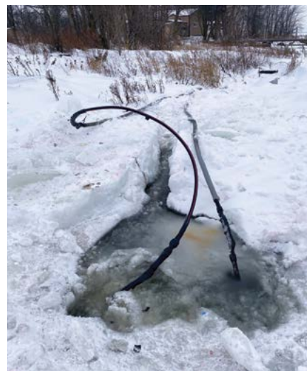
The fault that was located and repaired through the ice.
