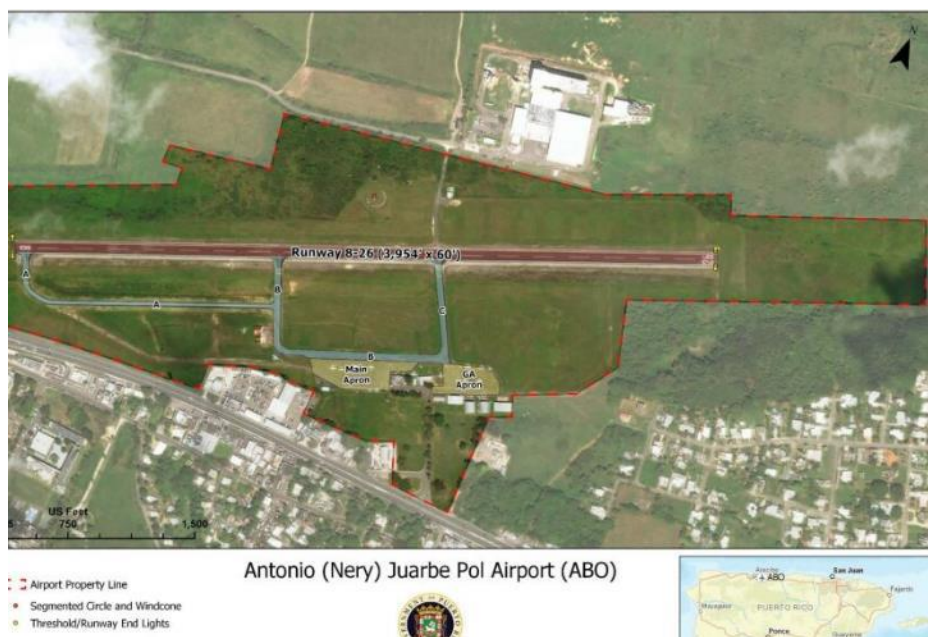
Figure 27. ABO Aerial Image
