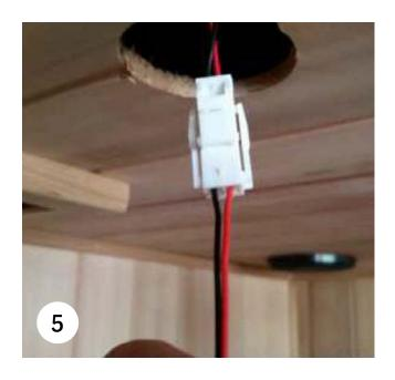
Connect the Red/Black cable coming out of the ceiling with the cable located on the back of the Medical Grade Chromotherapy device.
