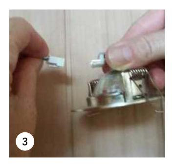
Disconnect the centre light from the Blue/White cable's connector. Push the Blue/White cable back up into the roof.
