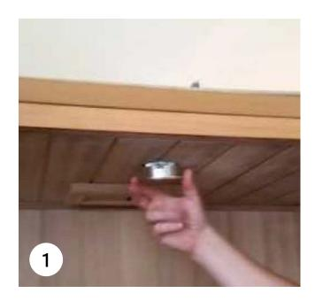
Using either your fingertips or a flathead screwdriver, slowly remove the centre Standard Chromotherapy light from the ceiling. Be careful of the spring coiled latches when removing the light, as they can act like a mousetrap and snap your fingers.
