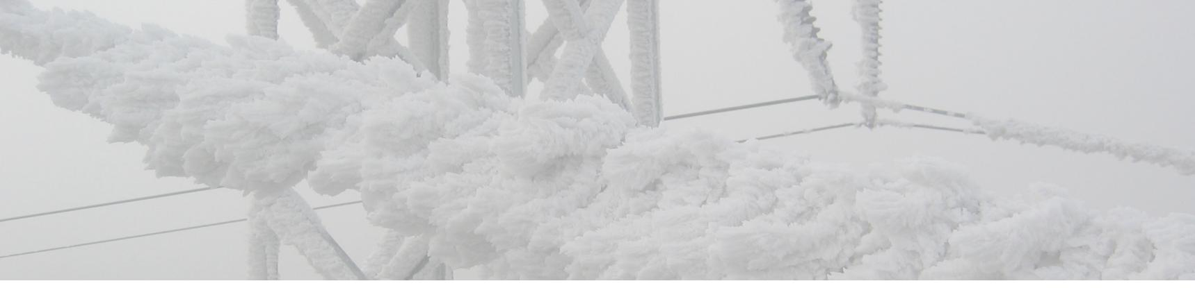
In-cloud icing, a particularly dense form, increases the tension of the conductor enough to encourage the utility to melt the ice. Photo: Gerhard Biedenbach, LineVision.
