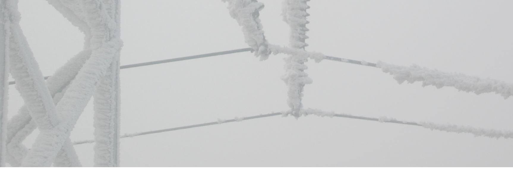
Ice has dropped in the left span but is still available on the right span. Suspension insulator swings to balance the tension. That decreases sag in the left-hand span and increases sag even more in the right-hand span. Photo: Gerhard Biedenbach, LineVision.
