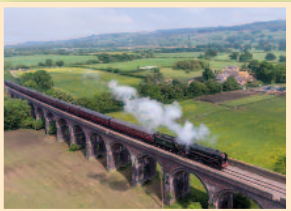
Stanway Viaduct 15 arches, 42 feet above the valley floor
