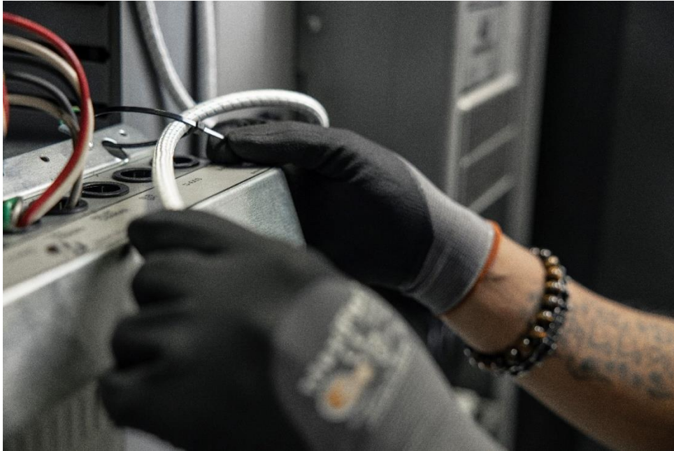
Figure 11 Securely fastening the FlexRope using the provided cable tie inside an electrical panel
