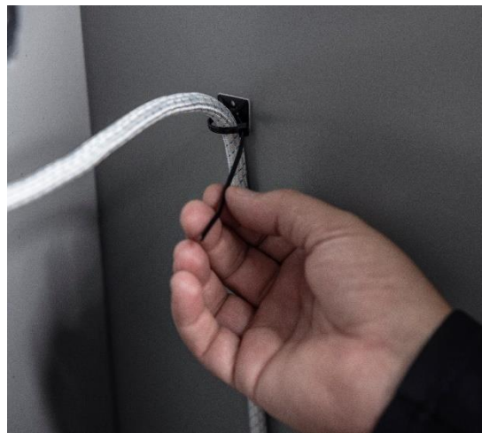
Figure 13 Pass the FlexRope through prepared cable tie and tighten
