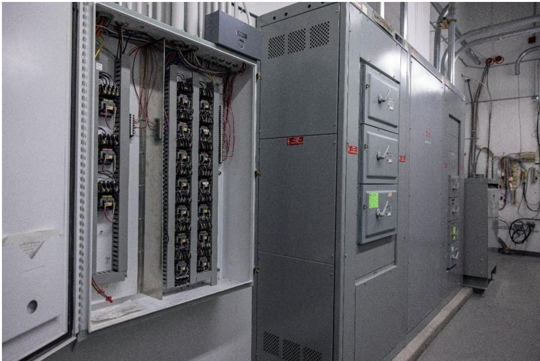
Figure 1 Example of a Relay Panel
