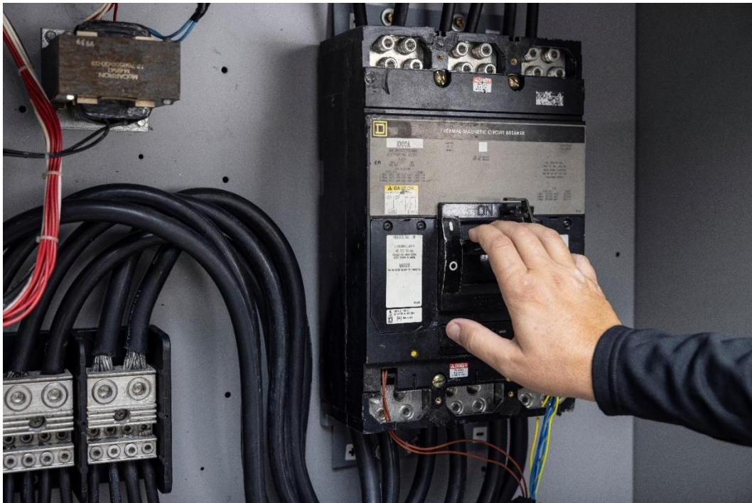
Figure 10 Ensure the electrical panel is de-energized before commencing any activity
