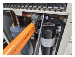
Figure 16 Connect Self-Sealing Coupling
