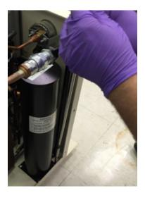
Figure 14 Install Adsorber
