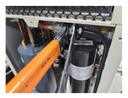
Figure 9 Disconnect Self-Sealing Coupling
