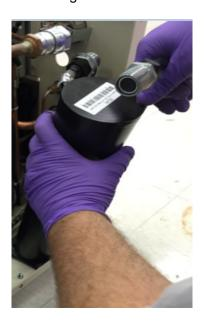
Figure 12 Remove Adsorber
