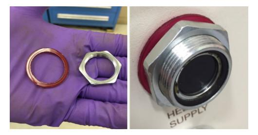
Figure 15 Install Supply Coupling Washer and Locknut
