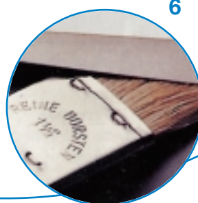
6 Longitudinal seam closed with special solvent-based adhesive
