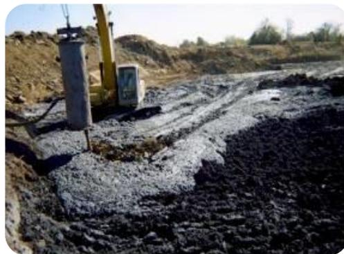
IKON excavated and handled over 110,000-cubic yards of onsite soil to provide a cover system (cap) over the on-site landfill. The footprint of the cap was expanded twice during the project to handle the excess soils from the impacted areas. The project also included the
