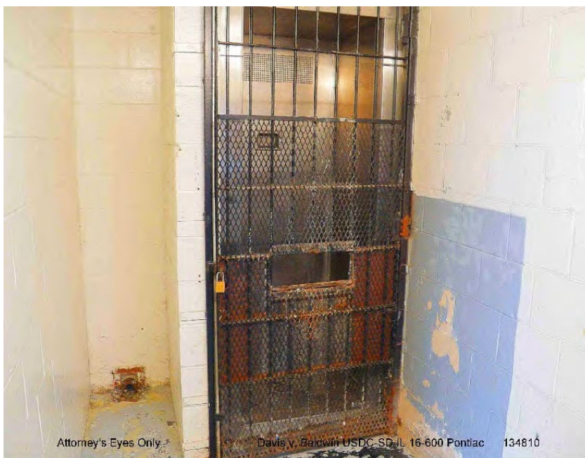
SHOWER, NORTH HOUSE 94
