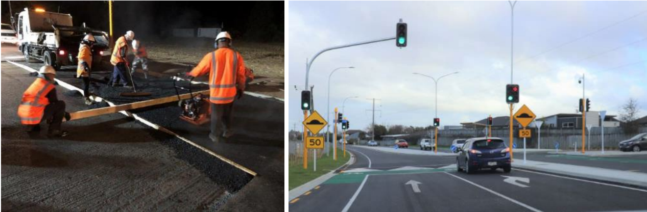
Figure 3.4. Construction of asphalt raised safety platform at Thomas/Gordonton Intersection, and resulting intersection layout, Hamilton, New Zealand
