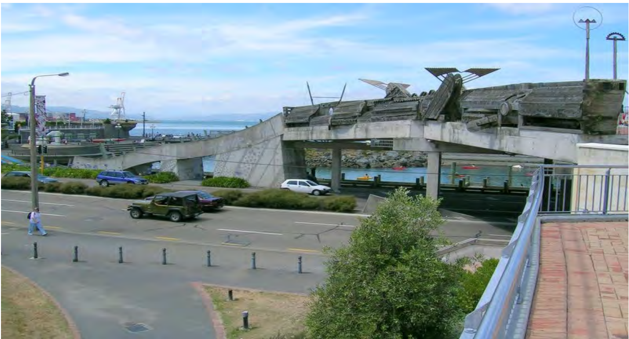
Figure B 41: Grade-separation for pedestrians and cyclists on a Movement Corridor/Connector Road (Wellington Waterfront, New Zealand)
