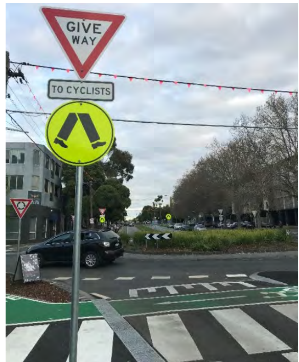
Figure B 12: Example of a roundabout with protected bicycle (and pedestrian) facilities (Melbourne suburb of Port Phillip)
