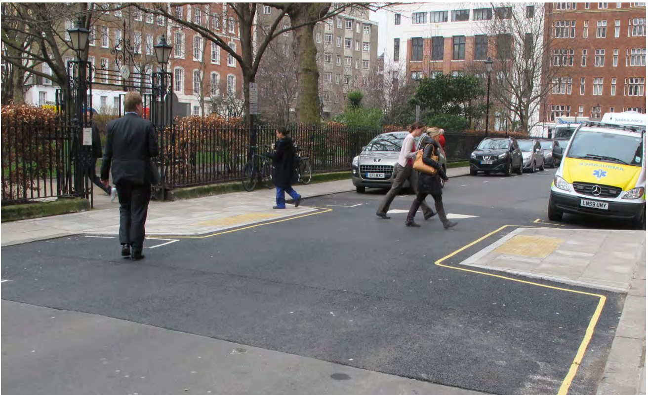
Figure 4.17: Kerb blisters with safety platforms in a 20 mph city street in London
