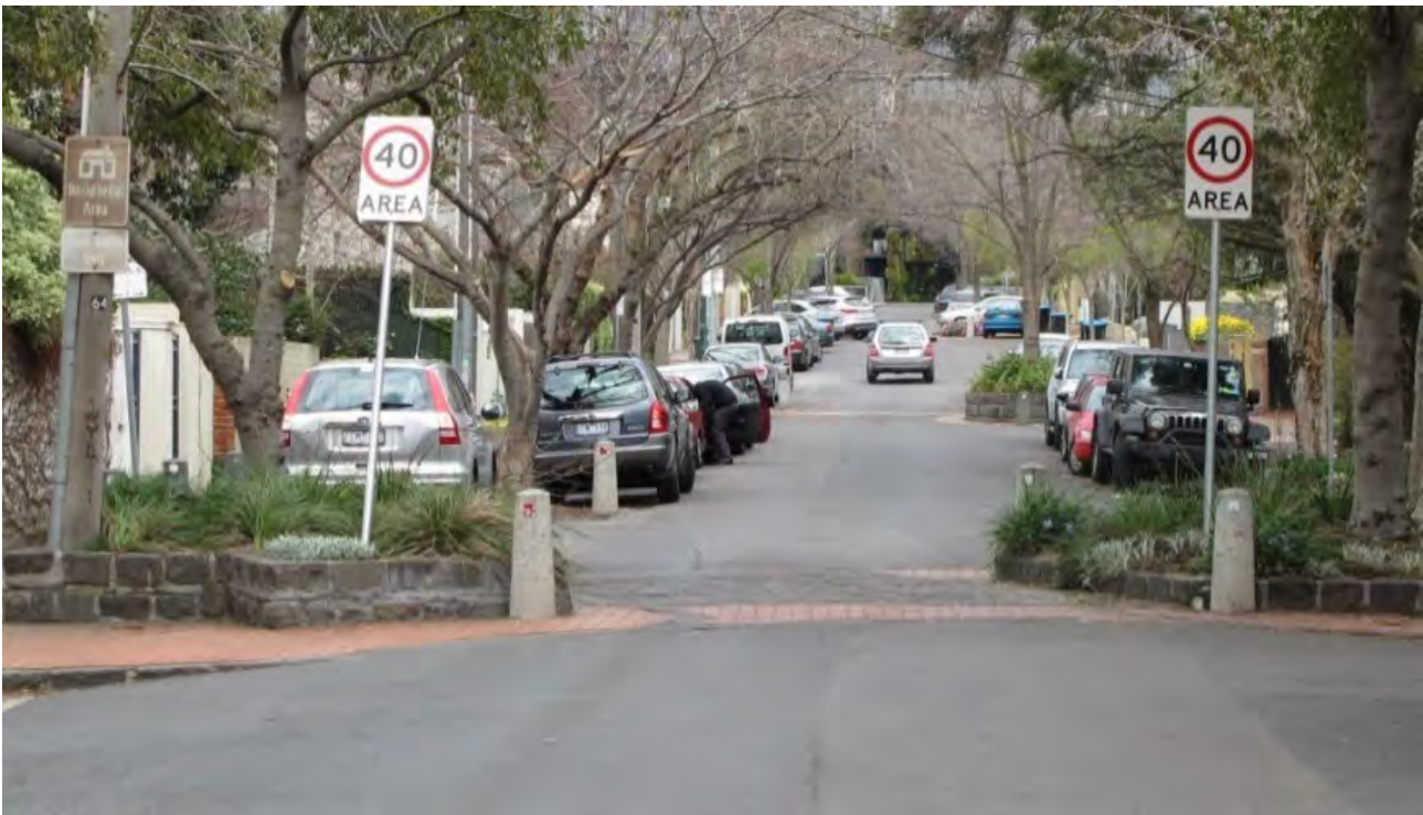
Figure B 27: Surface texture and colour, used in combination with horizontal deflection and kerb outstands (Melbourne suburb of South Yarra)
