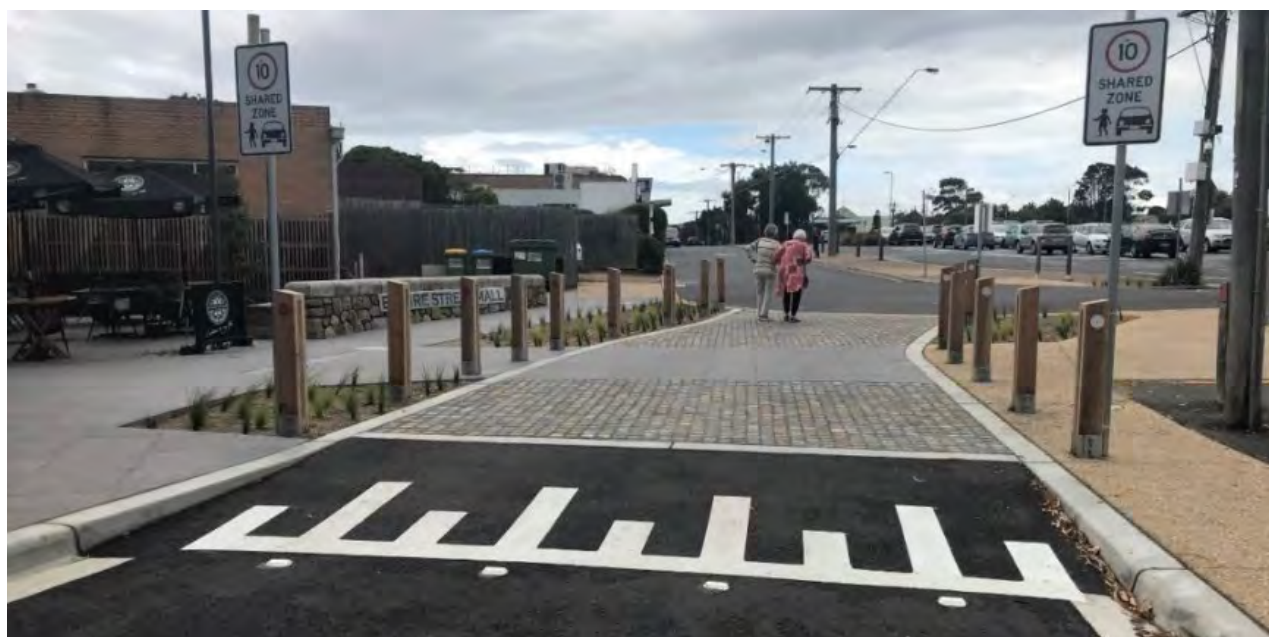
Figure B 28: Local Street shared space (10 km/h) together with speed platform, horizontal deflection and street plantings (Mornington, Victoria)
