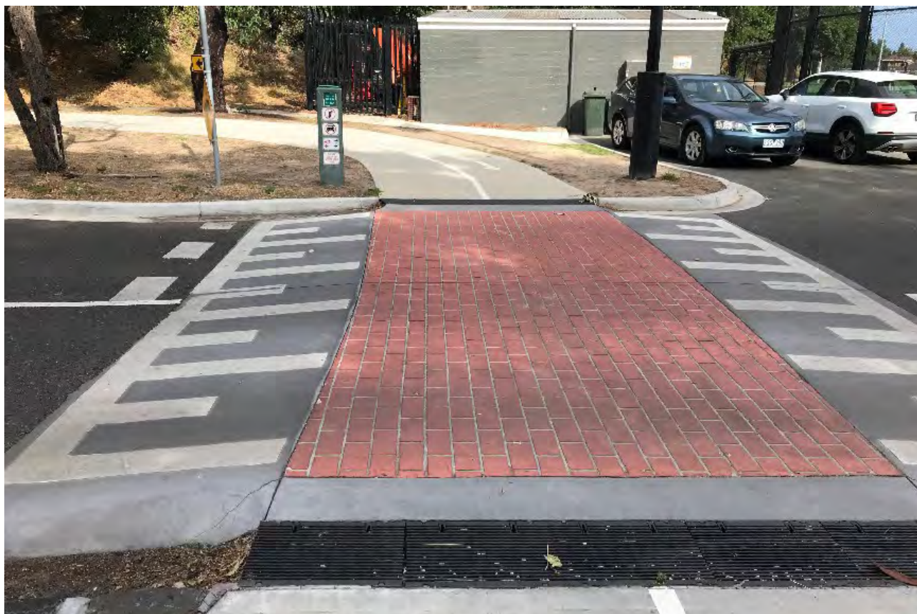
Figure B 32: Speed platform to moderate vehicle speeds where cycle paths meet minor side-streets and car-park access roads
