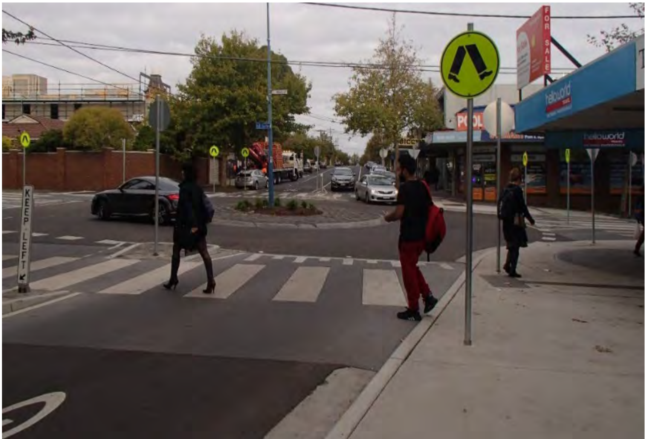
Figure 4.31: Roundabout with wombat crossings to cater for pedestrian movements – City of Bayside, Victoria
