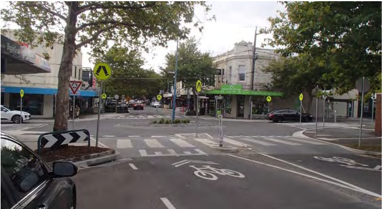
Figure B 18: Example of shared-use cyclists and general traffic lane, integrated with roundabout and wombat crossings (Church Street, Brighton, Victoria)
