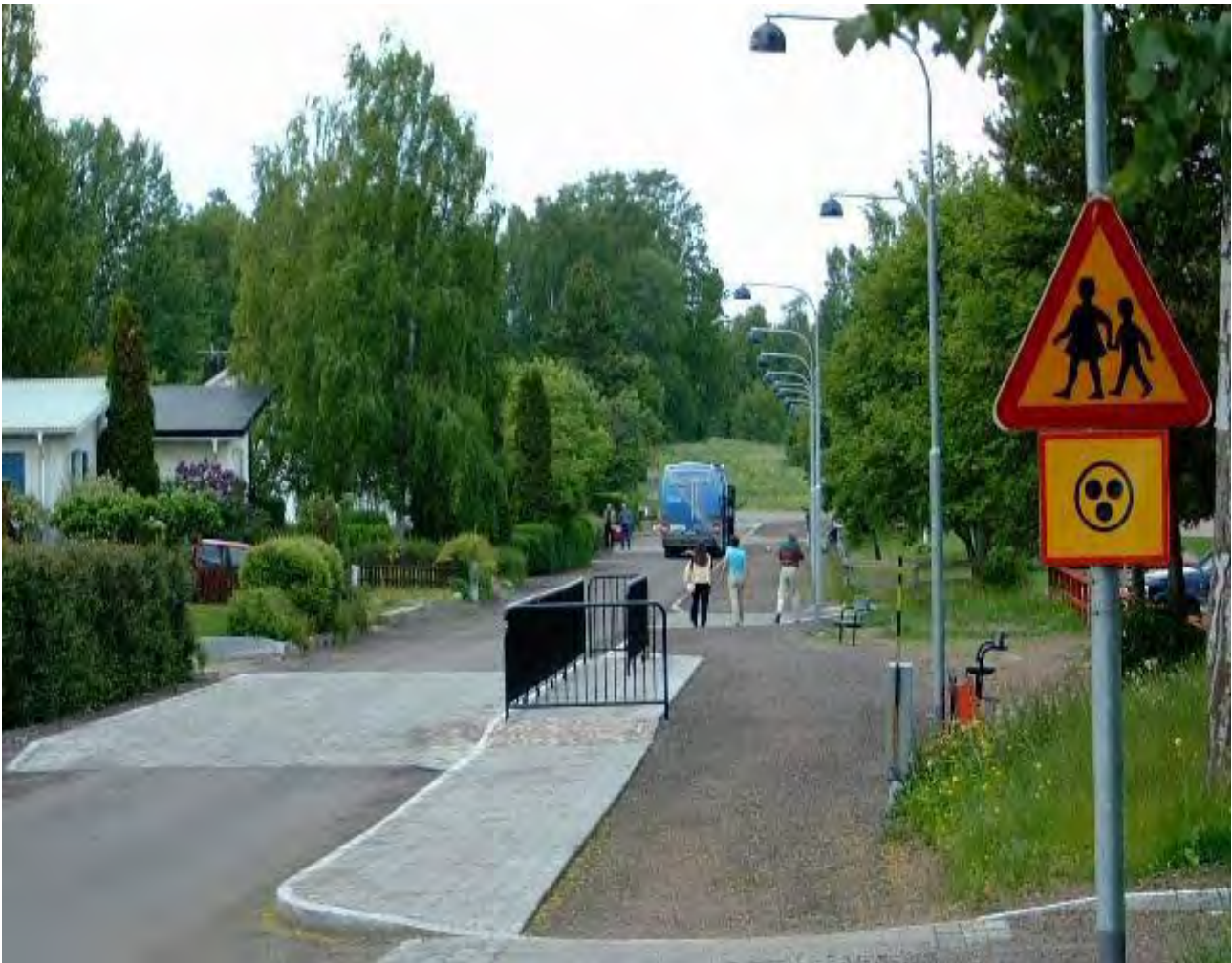
Figure B 26: Road narrowing at local streets bus stop in Sweden to prevent overtaking by general traffic
