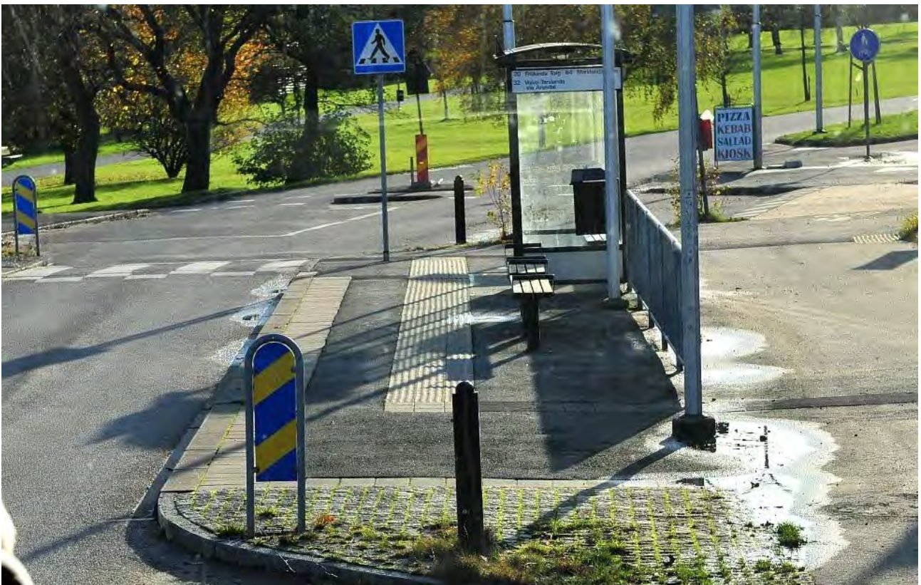
Figure 4.51: Road narrowing at Local Streets bus stop in Gothenburg, Sweden, to prevent overtaking by general traffic
