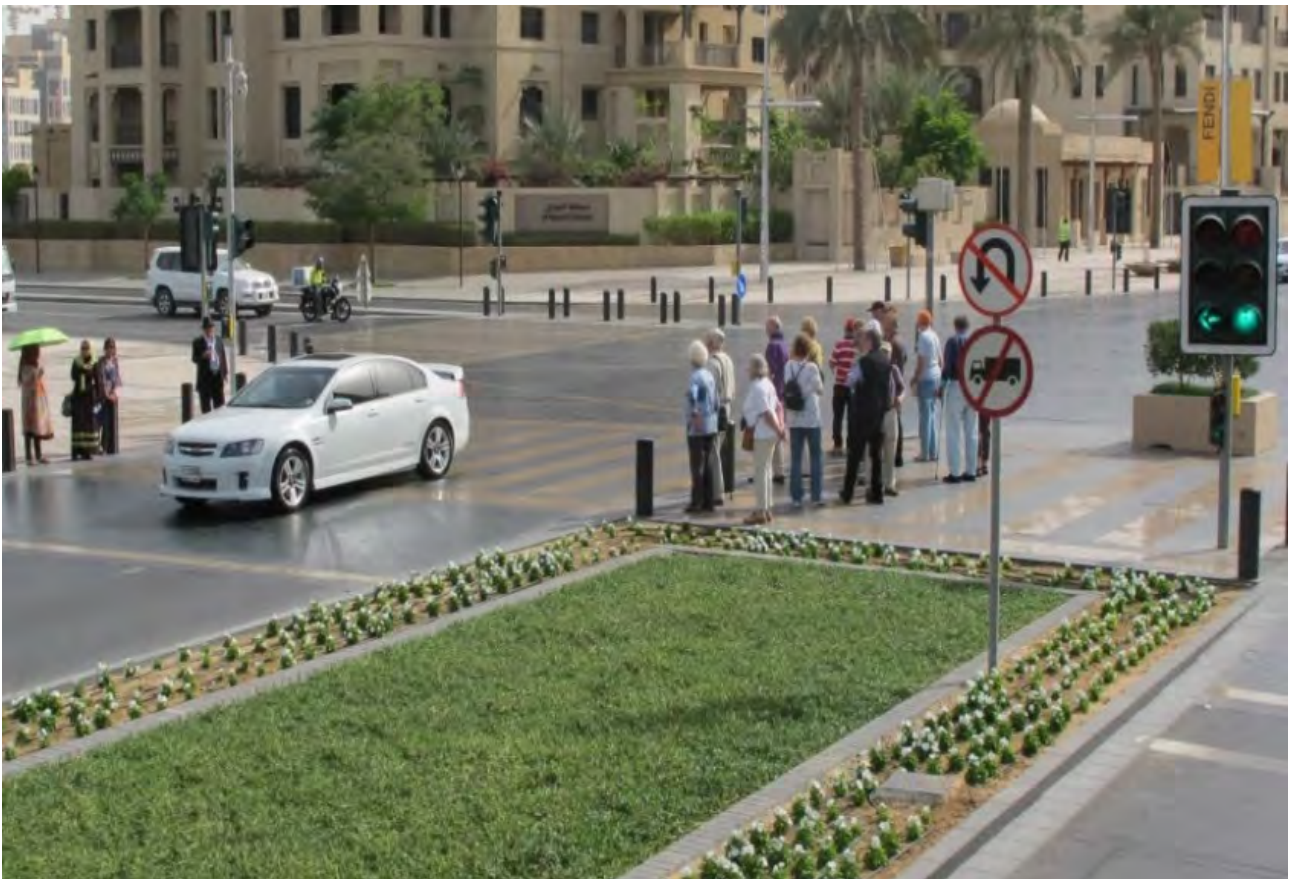
Figure 4.5: Raised signalised intersection in Dubai (many such intersections are equipped with Red Light and Speed Cameras operating on all approaches)
