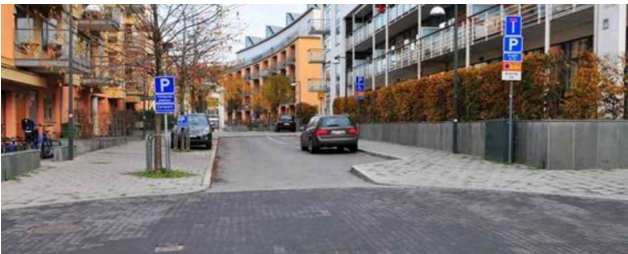
Figure 4.22: 30 km/h speed limit in combination with textured surfacing and single lane approaches suburb of Hammarby Sjöstad, Stockholm
