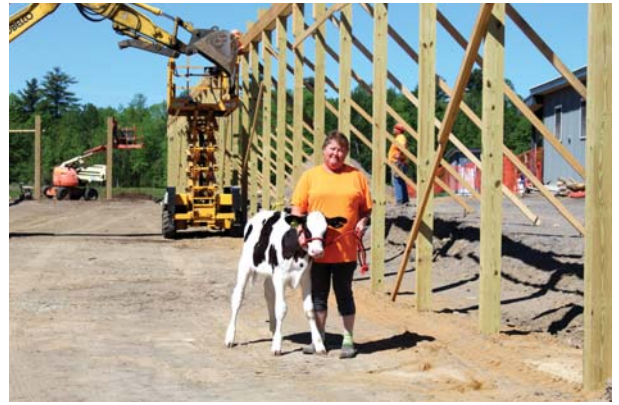
Bethann Buskey poses with a calf amid the barn construction on May 24, 2021.
