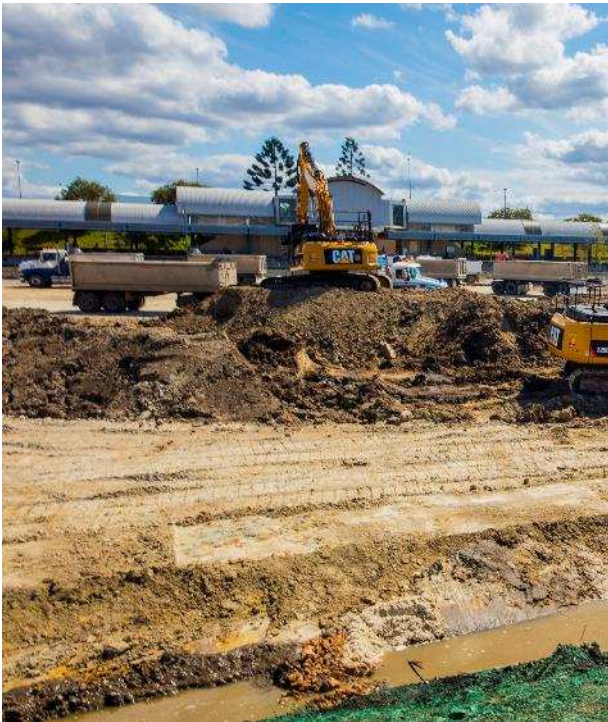
Work at Helensvale.
