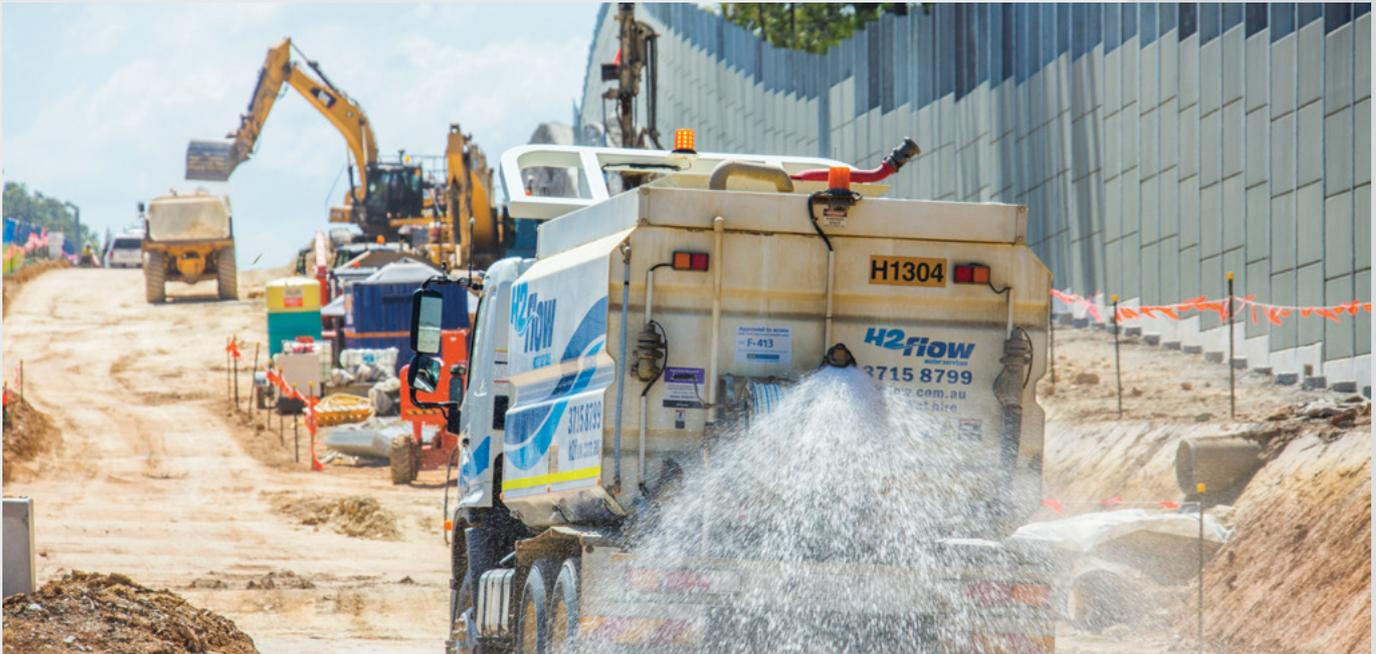
MAJOR EARTHWORKS ARE NEARING COMPLETION. DUST SUPPRESSION USING WATER TRUCKS.
