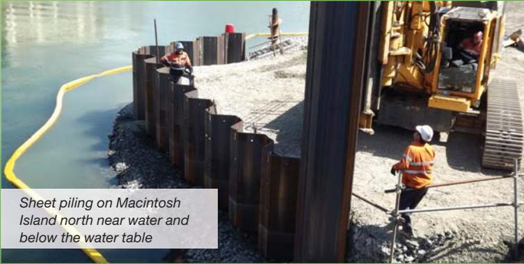
Sheet piling on Macintosh Island north near water and below the water table
