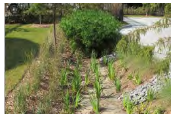
Bioswales capture stormwater runoff, helping it to absorb into the ground and clean the water.
