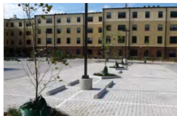
Pervious paving allows water to infiltrate on a site level. Because different areas have different soil composition, design needs to be site specific.
