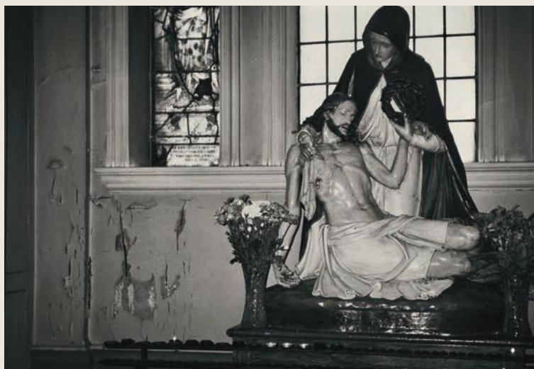
Damp had caused major deterioration to the church walls and ceilings.
