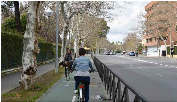
Bike lanes were installed at sidewalk level for greater protection.
