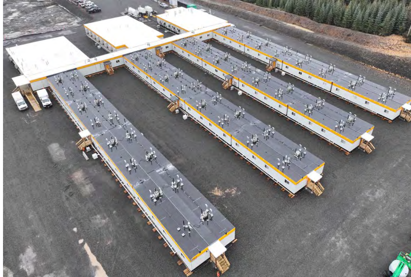
CAMP 11 WORK AREA
