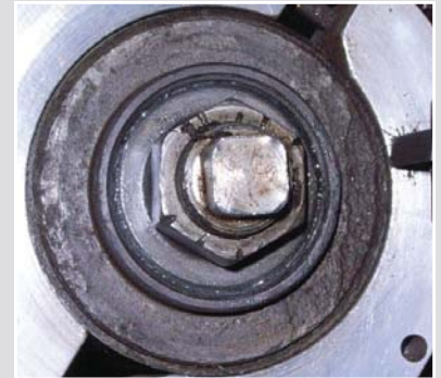
Access Fitting before re-facing
