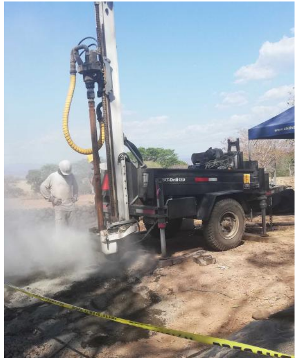
THE TEAM WORKS ON DRILLING A BOREHOLE.
