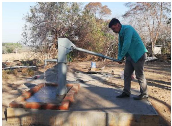
THE WELL IS COMPLETE!
