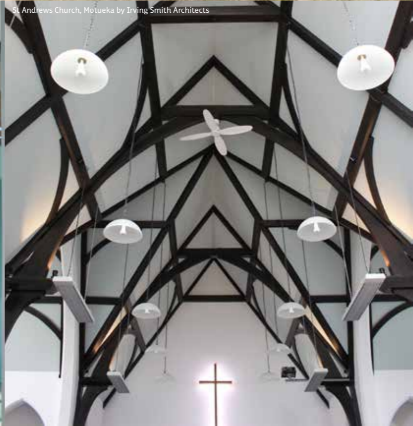
St Andrews Church, Motueka by Irving Smith Architects
