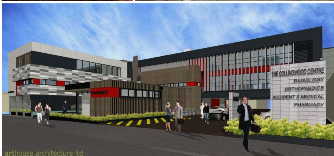
Above: architect Jorgen Andersen surveys the exterior during construction; terracotta tiling echoes the pattern of DNA; Nelson Radiology's $700,000 CT scanner being hoisted onto the first floor; architect's impression of the finished building
