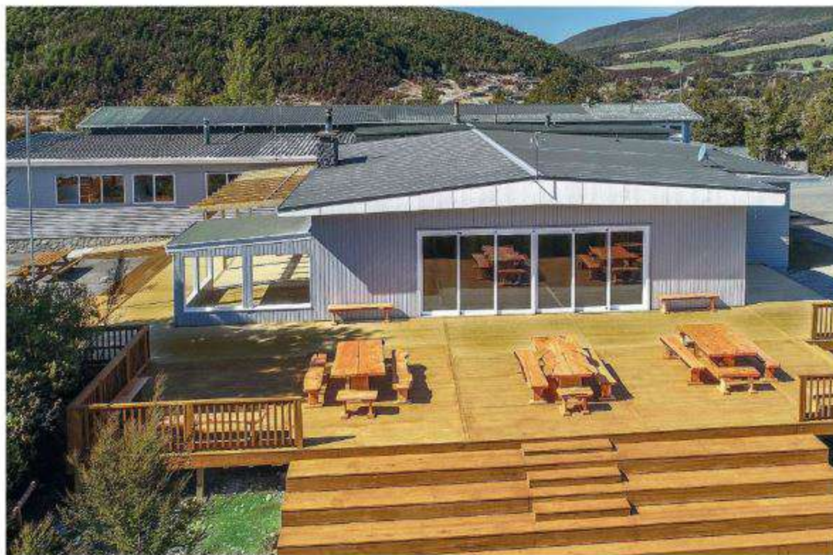
The newly refurbished Rotoiti Lodge.
