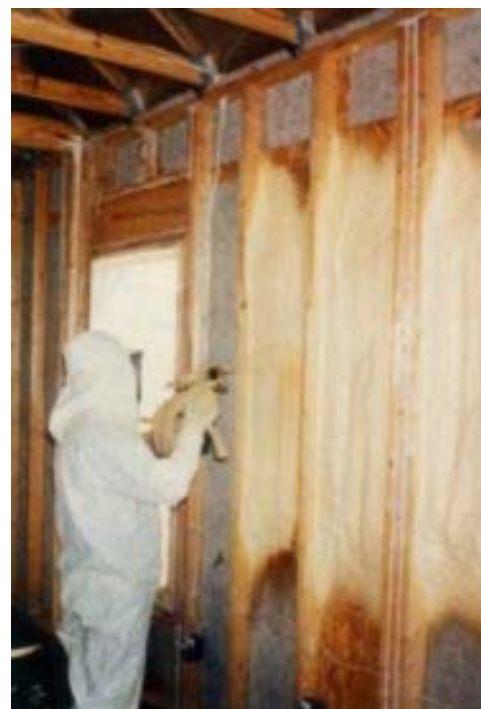
Application of NCFI spray insulation to stud wall cavity.
