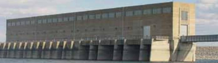
The purpose of the Intake Structure is to house the necessary hoisting equipment, gates and auxiliary equipment for the eight water tunnels. Five of the tunnels are for power generation and three are for regulating water releases.
