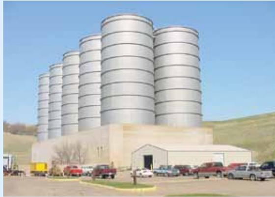
The purpose of the surge tanks is to absorb the shock from the sudden stopping of water flow by the wicket gates. The surge tanks are made of welded steel plate.
