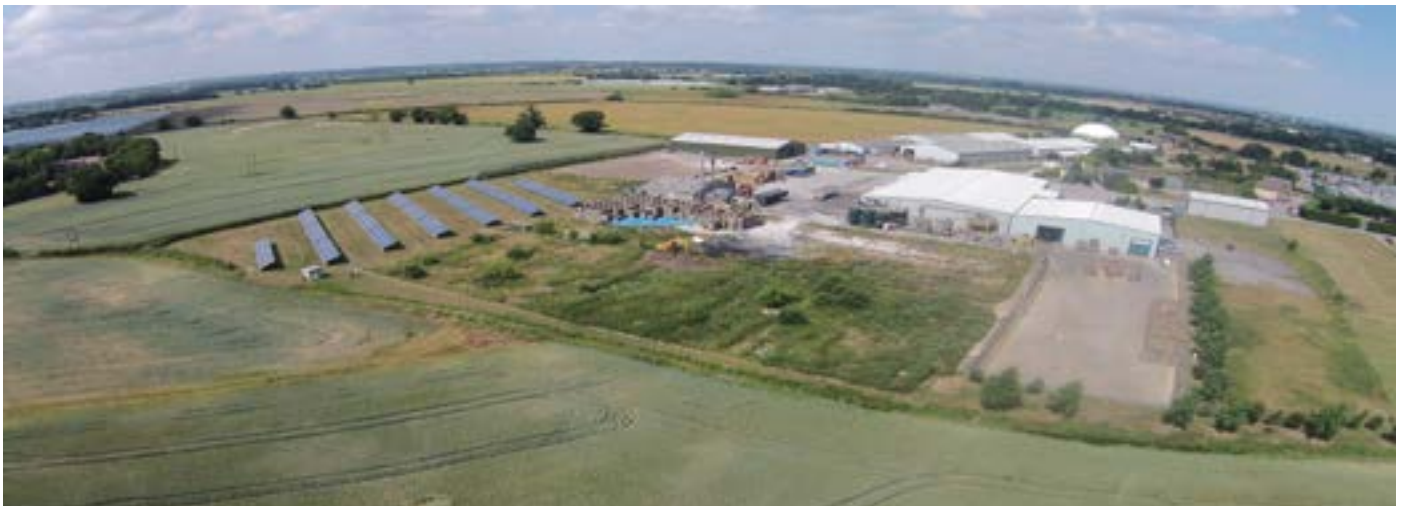
The site at Plaxton Bridge
