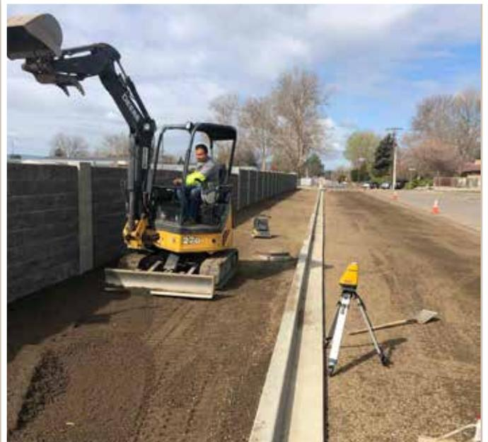
Above, Sal is making sidewalk prep look easy! To the right is the new half of the street prepped. The developer was also required to put in a 10 foot wide sidewalk, storm drainage, curb and gutter for his side. The other side has somehow survived for years and likely will for many more! Below is the almost finished project showing both sides of the street.
