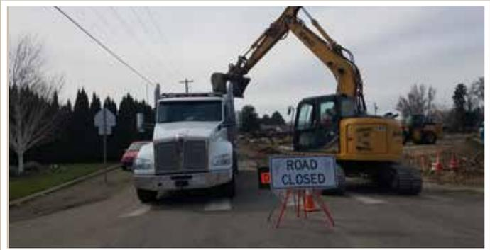
Final stages of a small subdivision going in. The City required that the half of the road next to the development be rebuilt to current standards. Hard for this farm boy to get his head around since the other side of the road is developed and will never be rebuilt to match. We also took out 4" of asphalt, replacing it with 3" and added a lot more gravel underneath since the existing only had 4" to 6".
