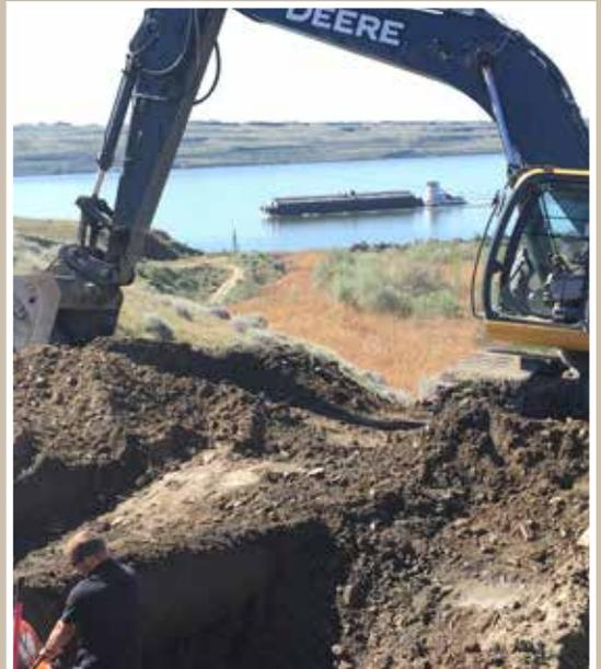
What a picture! Here Robert and crew are working on a steep hill doing an emergency 30" steel leak repair for a long time customer. So cool to catch the barge at just the right time!
