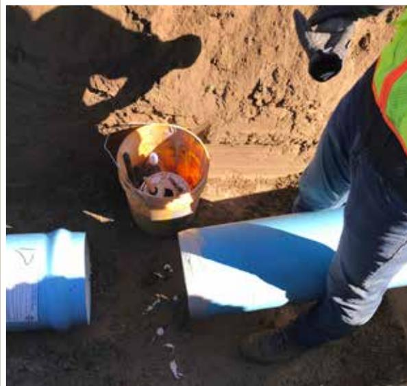
The position of pipe layer is extremely critical to the long term success of the pipeline. Here you see the tools of the trade and a pipe that is properly lubed and ready to be slid into place.
