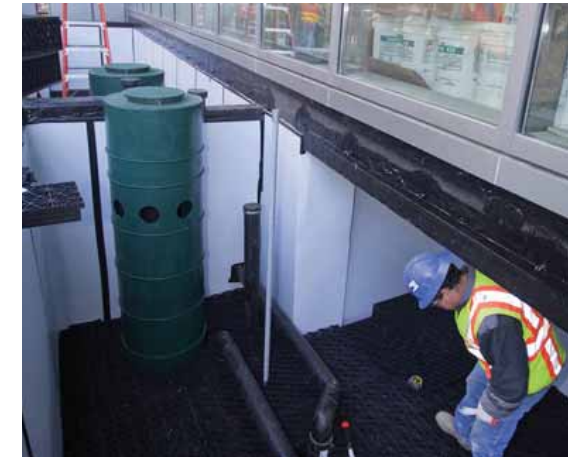
Exterior Tidal Flow Wetland Cells- Installation of Underdrain
