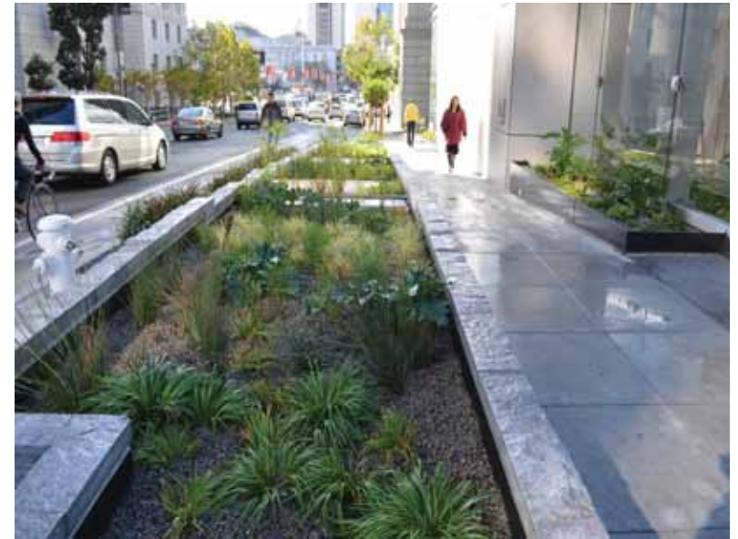
Exterior of 525 Golden Gate Avenue with Vertical Flow Wetland Cell
