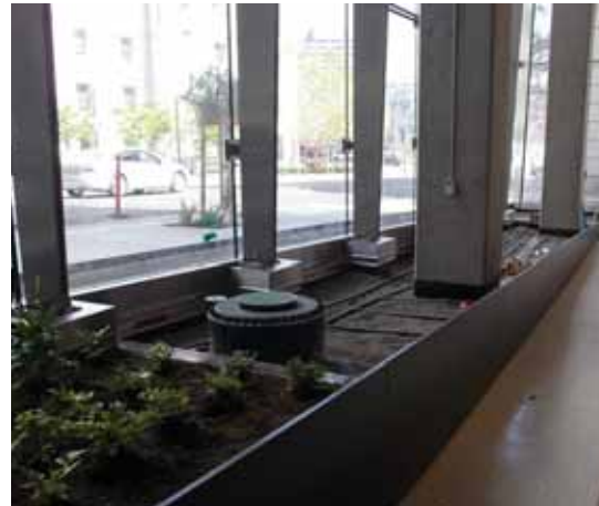
Final Construction Phase - Interior Vertical Flow Wetland Cells
