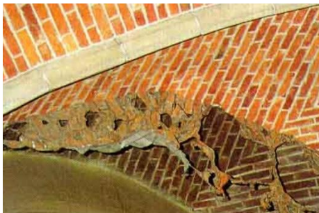
Cleaning of bricks
