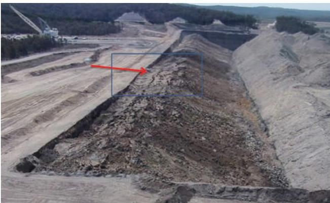
**FIG 6** – Case study 1 – muck pile profile for dragline access from the middle of the shot.
