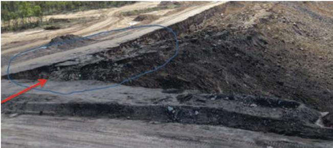
**FIG 5** – Case study 1 – blast result showing the muck pile profile for the dragline’s access to the shot. Arrow indicates the direction of access for the dragline.
