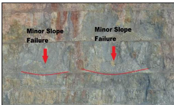
Figure 3. Minor slope failures at north-east section of the pit.
