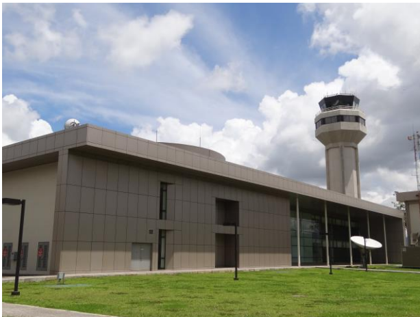
Trinidad & Tobago Civil Aviation Authority Facility
