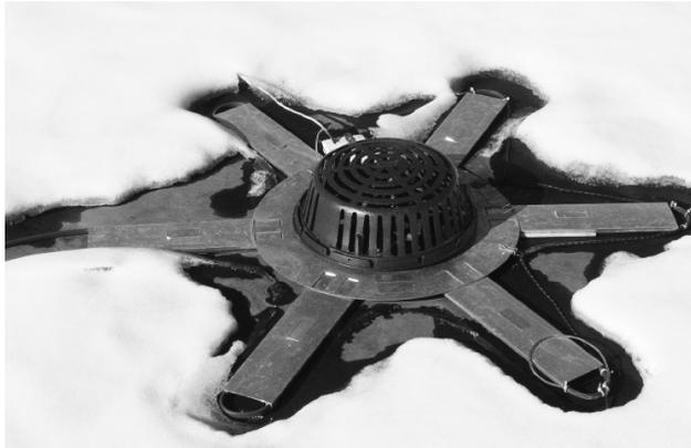
Figure 1. **Primary roof drainage. DT-RFDR-6: Flat Roof Drain Hub with 6 Rays**
