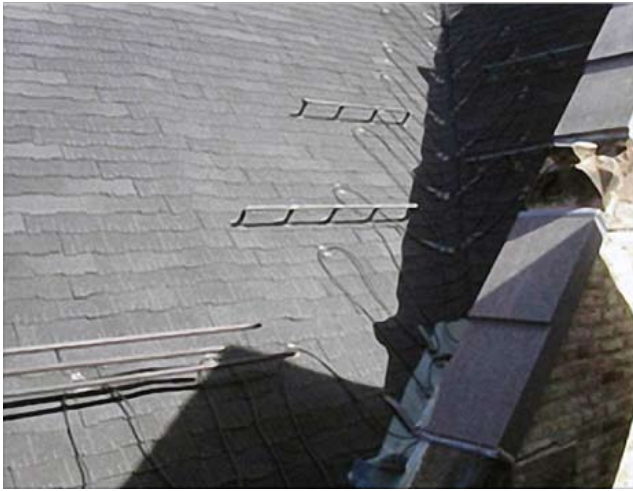
Delta-Therm deicing cable is installed behind the brick façade to create a heated drain path for snow melt water to follow.
