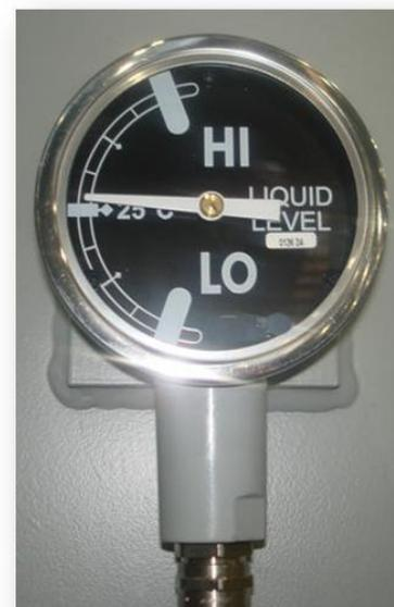
seam. The other possibility is that the transformer is lightly loaded but is installed in an extremely cold location. This is possible since insulating fluid not only expands with heat but also contracts proportionally in cold environments.
